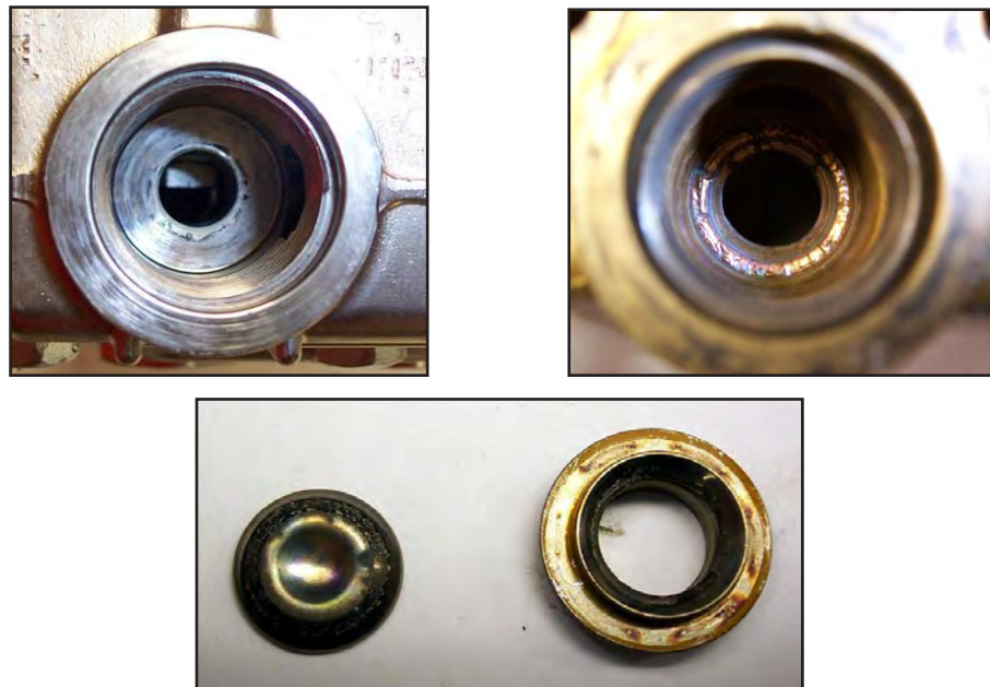
Figure 5-2. Inspect Manifold and Old Valves
